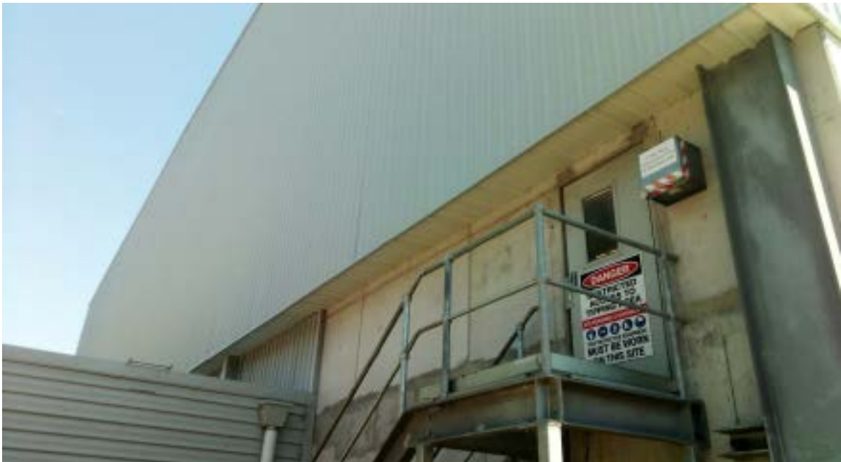
Figure 1- Sealed southern breezeway of the waste shed at the Terminal
