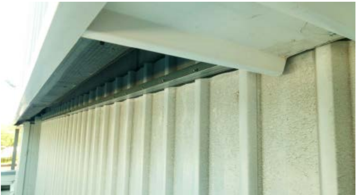
Figure-2 - Sealed South-eastern breezeway of waste shed at the Terminal
