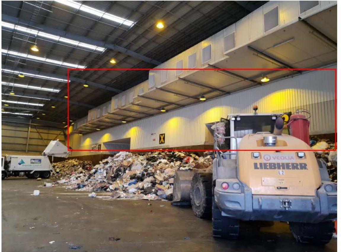
Figure 3 - A view of the completed sealing up of the gap opening between the interface of the waste floor and compactor pit areas at the Terminal
