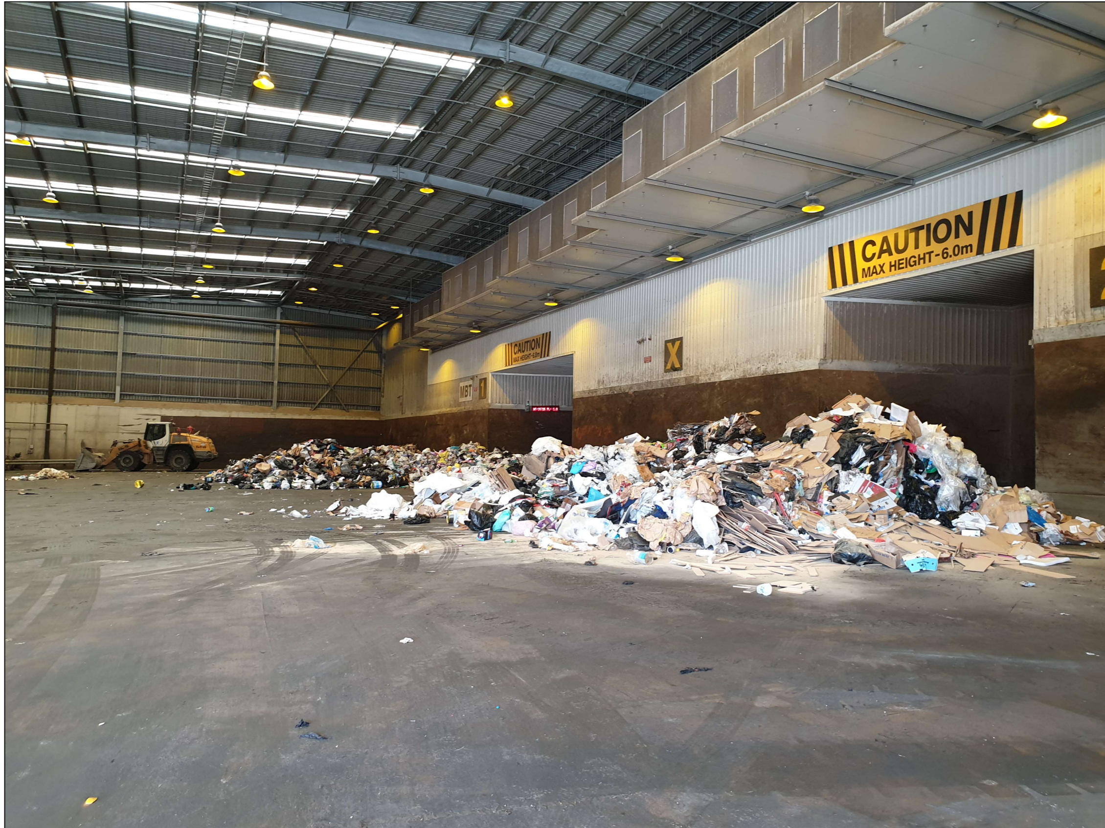
Photo 3 – The BTT Facility waste floor area as found on 10 April 2019
