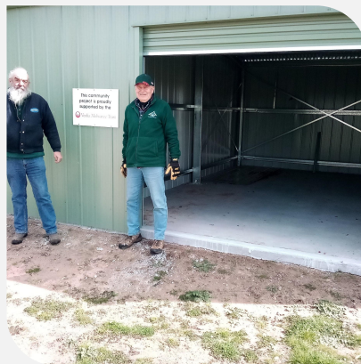
New catering and storage area at Tarago Showground
