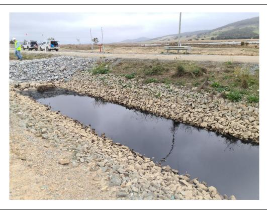
**Photo 2.6** – A view of the V-drain servicing the Maturation Pad at the MBT Facility: 24 March 2022
