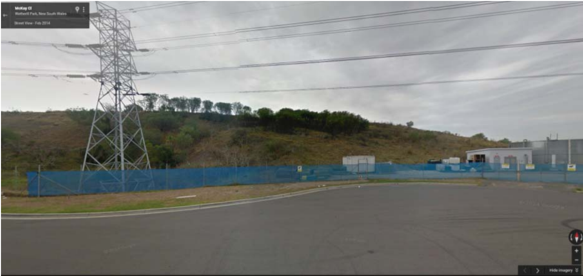
Figure 14.5: View north towards the Wetherill Park Resource Recovery Facility from McKay Close cul de sac (Source: Google Street View)
