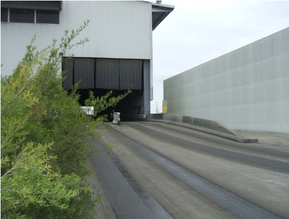
Figure 3 Uphill Incline to Transfer Building
