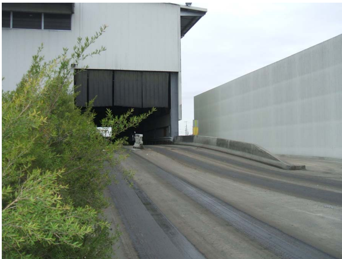
Figure 3 Up-ramp Leading into Transfer Facility
