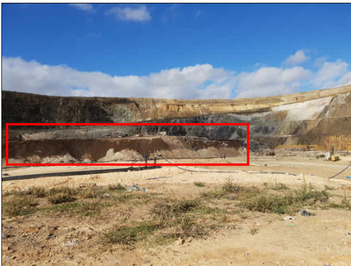
Photo 7.1 – Biofilter cover material applied on the active tipping face batter as occurred on 21 February 2019
