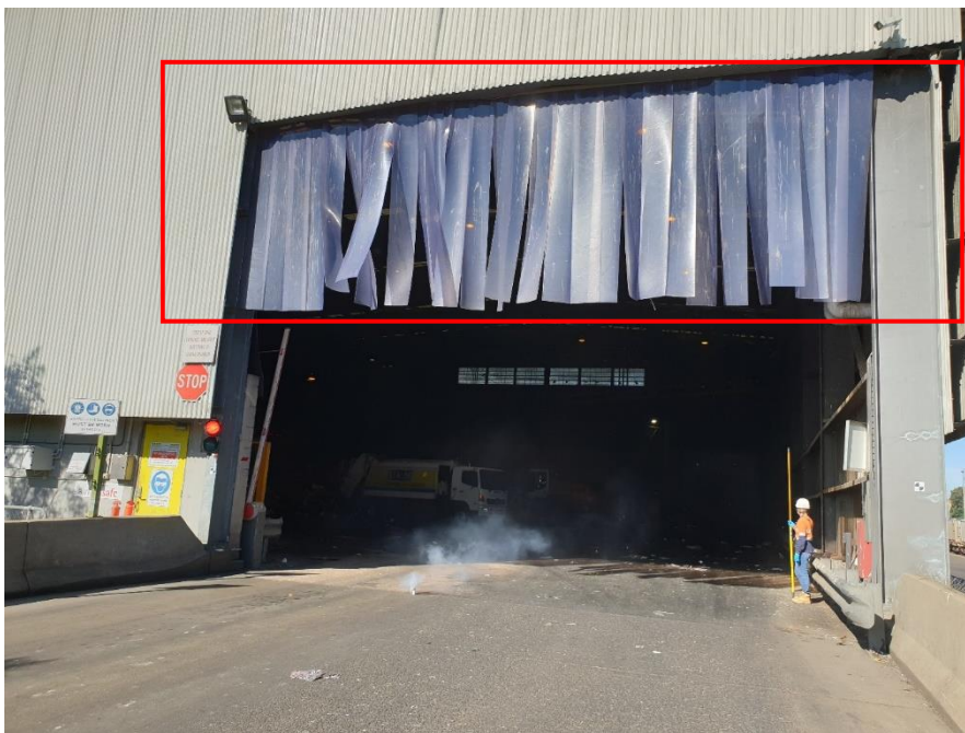
Photo 2.5 – A view of the truck entrance plastic strips during smoke testing on 6 May 2020
