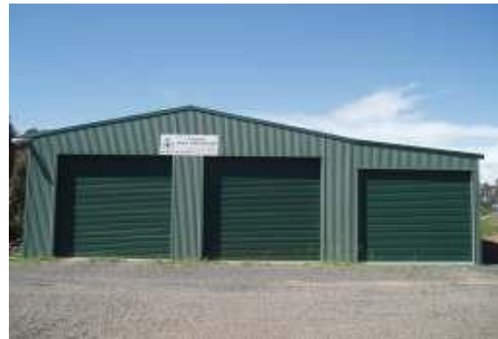
Extensions to the Gundry Rural Fire Shed provide vehicle storage and toilet and washing facilities
