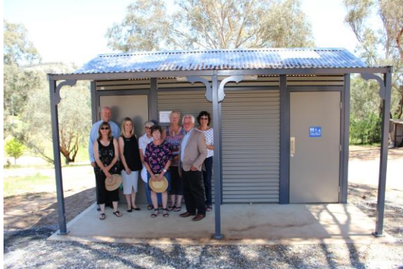
A new accessible toilet block constructed at Tuena
