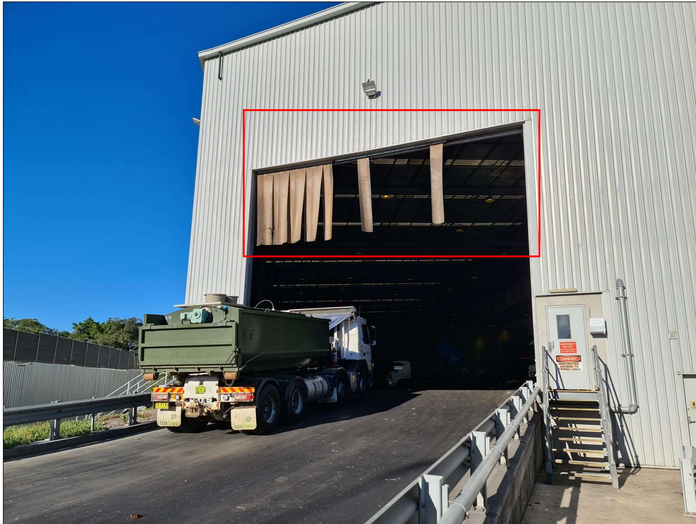
Photo 4 – A view of the truck entry point to the BTT Facility building: 14 May 2021 (Note The truck entrance plastics strips were found to be missing a few panels)
