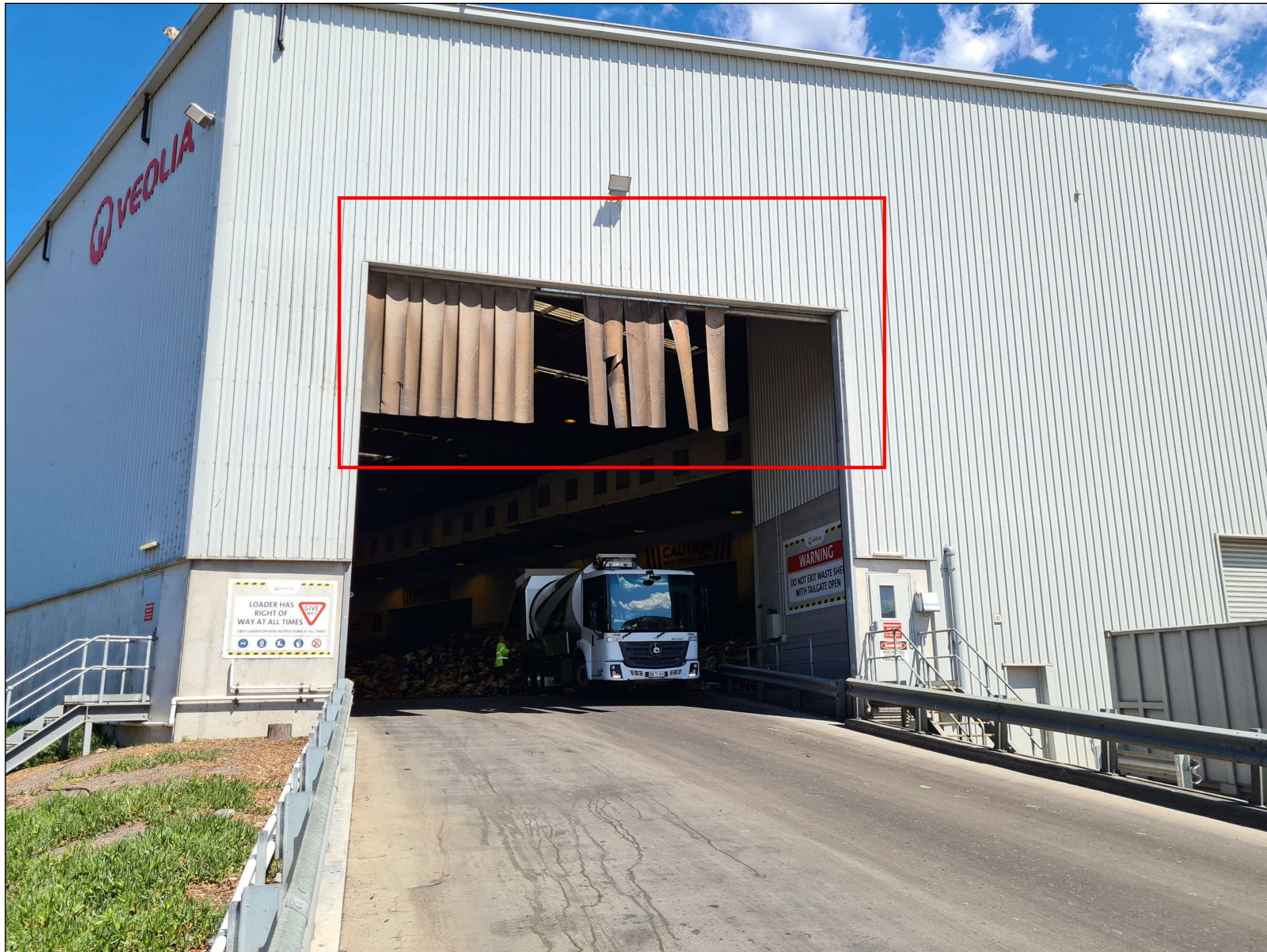
Photo 3 – The truck entrance plastics strips were found to be missing a few panels: 1 October 2020
