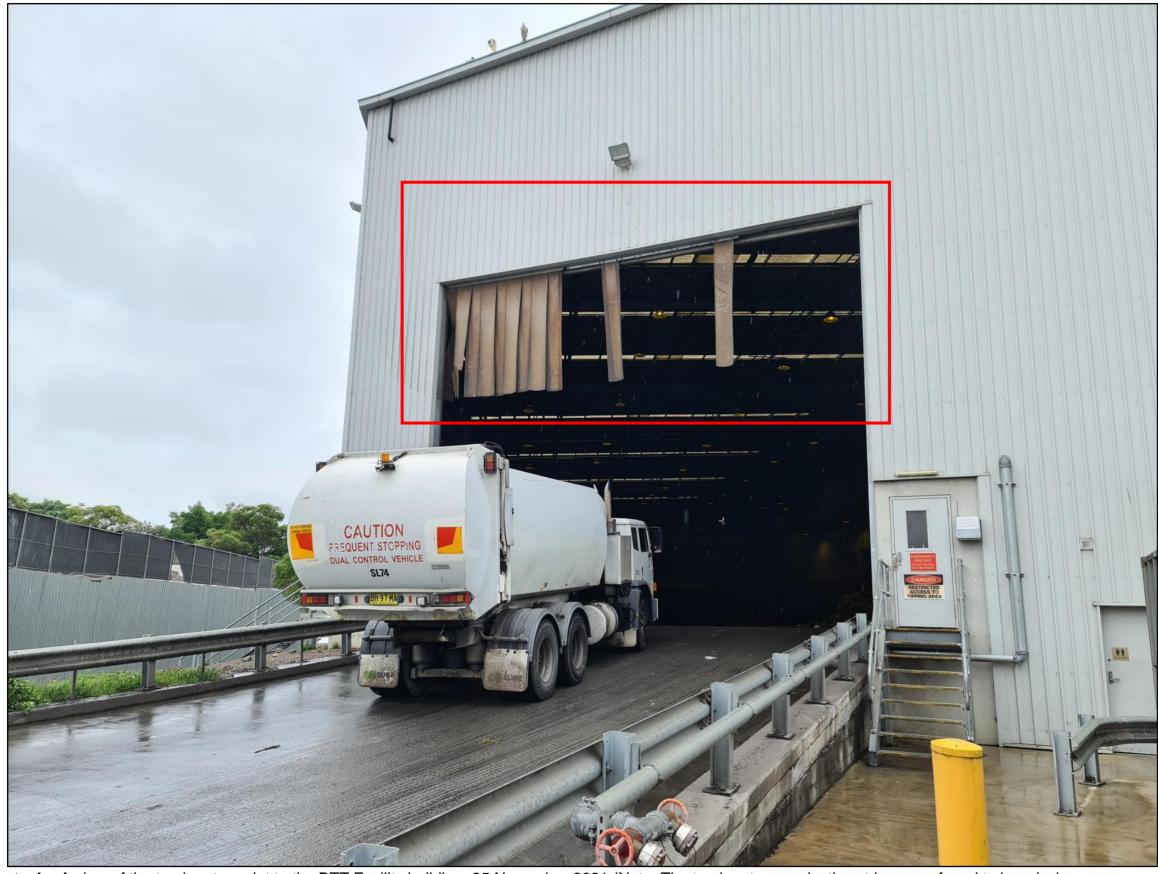
Photo 4 – A view of the truck entry point to the BTT Facility building: 25 November 2021 (Note: The truck entrance plastics strips were found to be missing some panels)
