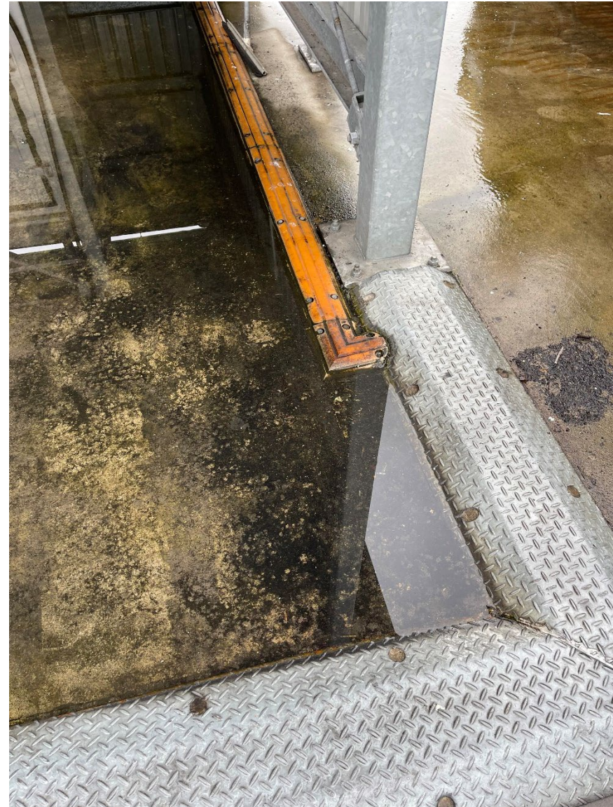
Figure F4. Stormwater ingress into fuel storage bund area.
