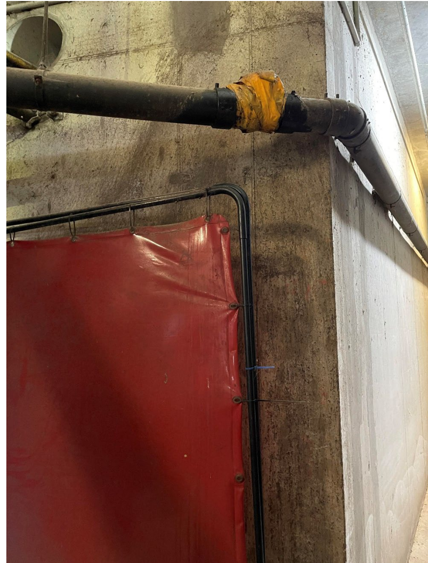
Figure F2. Poorly repaired and leaking leachate transfer line.
