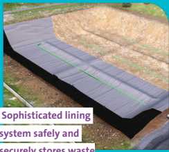
Water that comes into contact with waste is captured and treated
