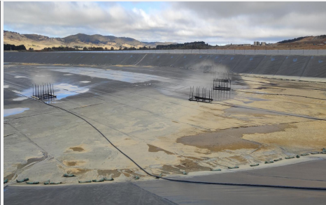
Coffer #2 2023 and start spray discharge for better evaporation
