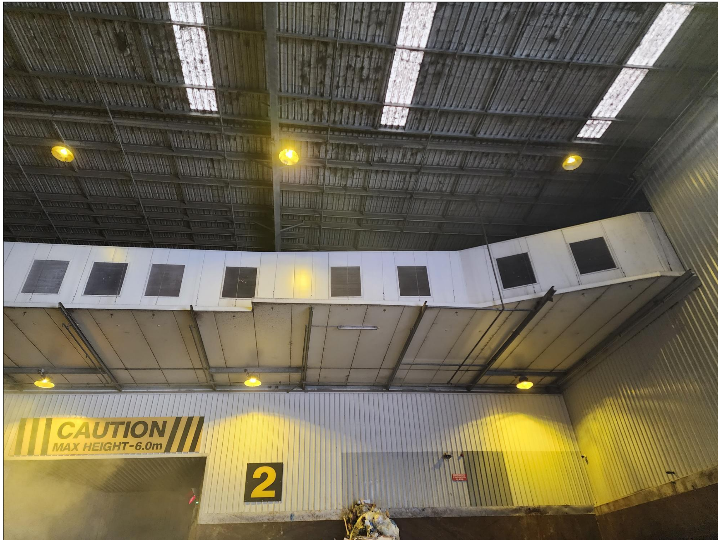
Photo 4 – A view of the ventilation collection points: 4 July 2023 (Note: The walls and collection grilles have been cleaned since the December 2022 Audit)
