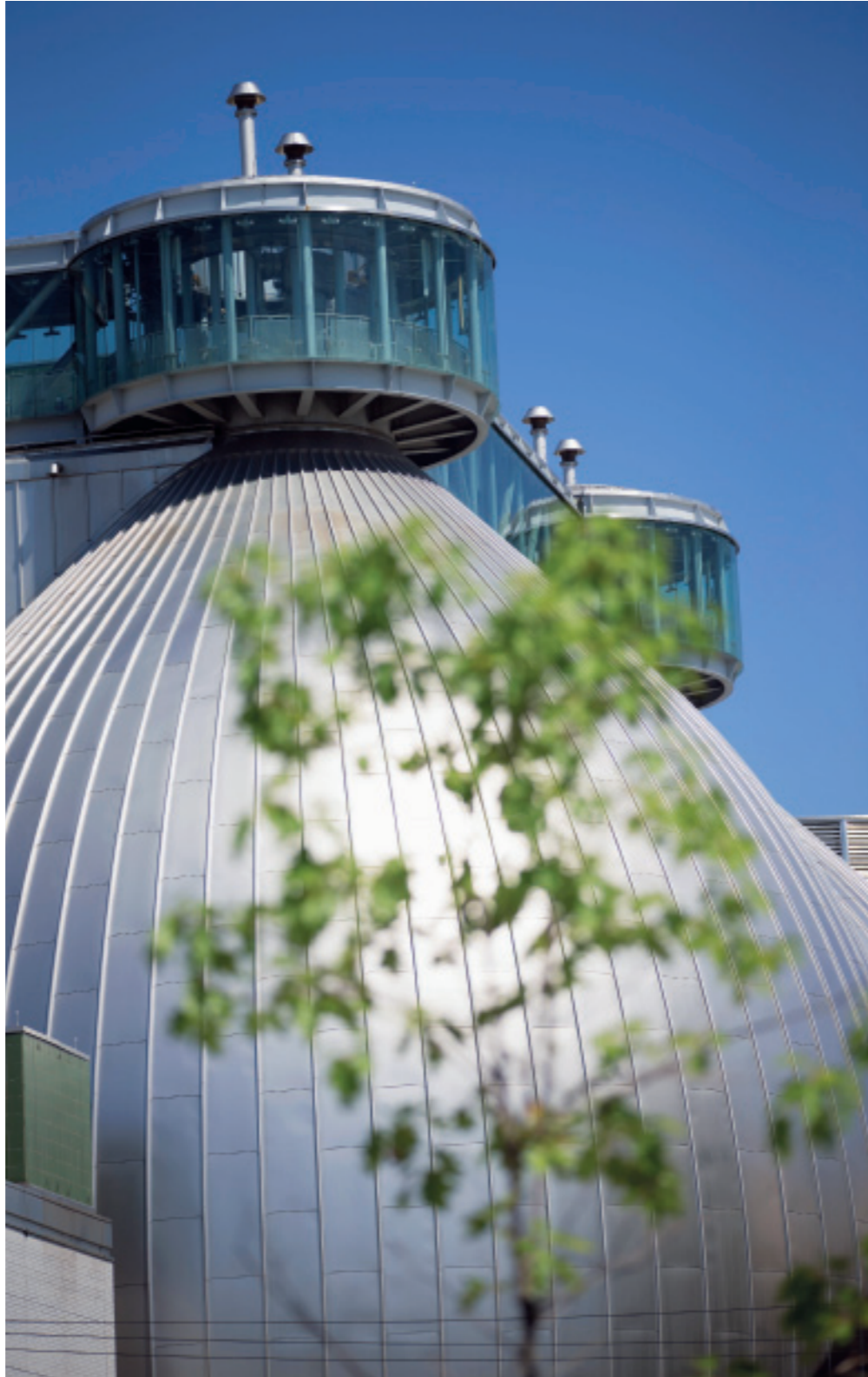
In Brooklyn, Newtown Creek is the largest of New York City's 14 wastewater treatment plants.
