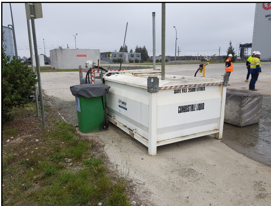
Photo 28: Self-bunded white Diesel tank (2,500 L) with Spill Kit next to it. 24/03/22
