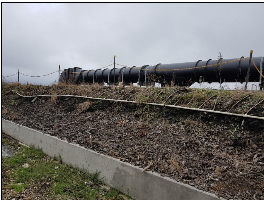
Photo 6: Biofilters #2 and #3 within the central portion of the site with weeds growing on the filter media. 24/03/22
