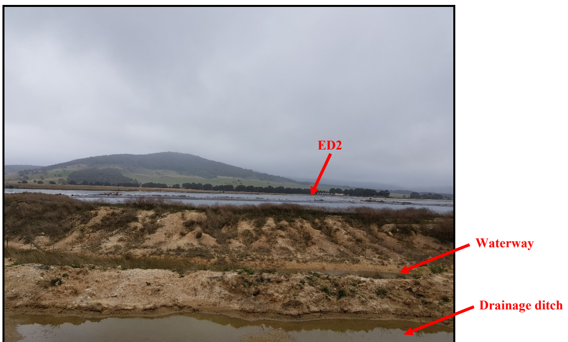
Photo 22: Looking north across a drainage ditch and the waterway with ED2 in the background. Some vegetation cover observed on the embankments in the foreground but erosion also evident on far embankment. 24/03/22
