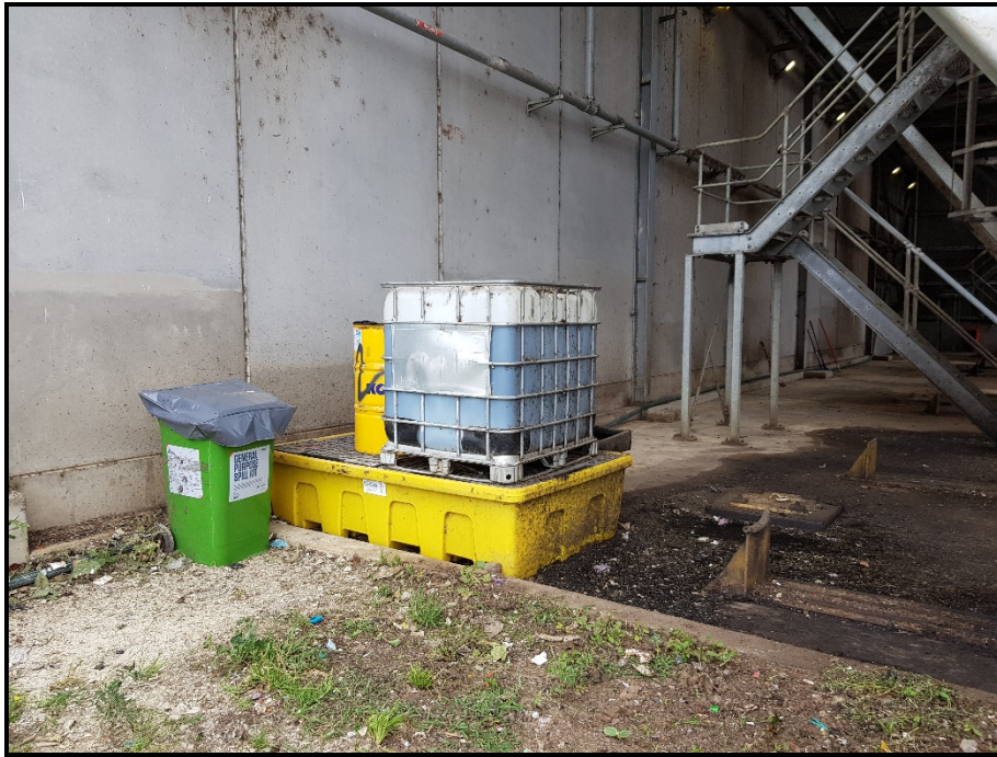
Photo 25: Bunded IBC containing waste oil with Spill Kit next to it. 24/03/22
