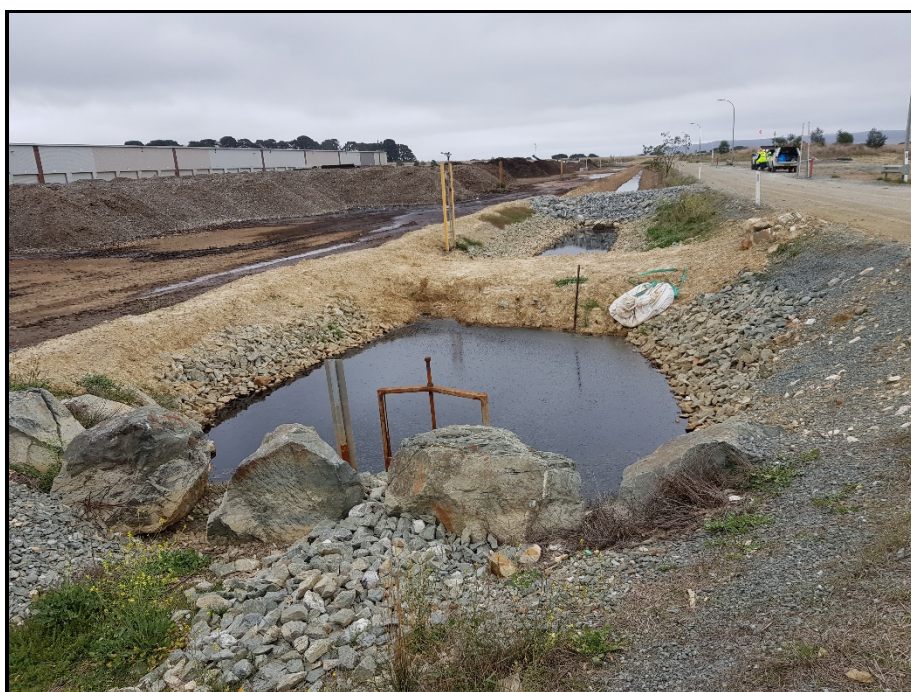
Photo 10: Looking west with the Fermentation Building and Maturation Pad on the left, the leachate drainage system that drains towards the leachate ponds located behind the photographer. 24/03/22
