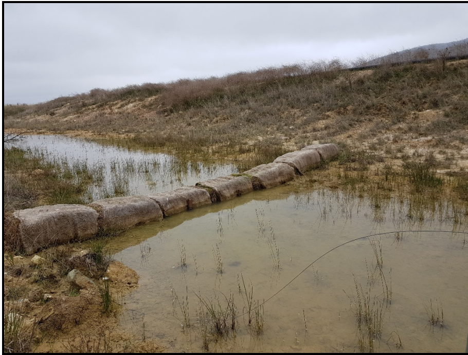
Photo 21: Sedimentation control in the form of hay bales in the waterway, upstream of EPA Point 8. Some vegetation cover observed on the embankment. 24/03/22
