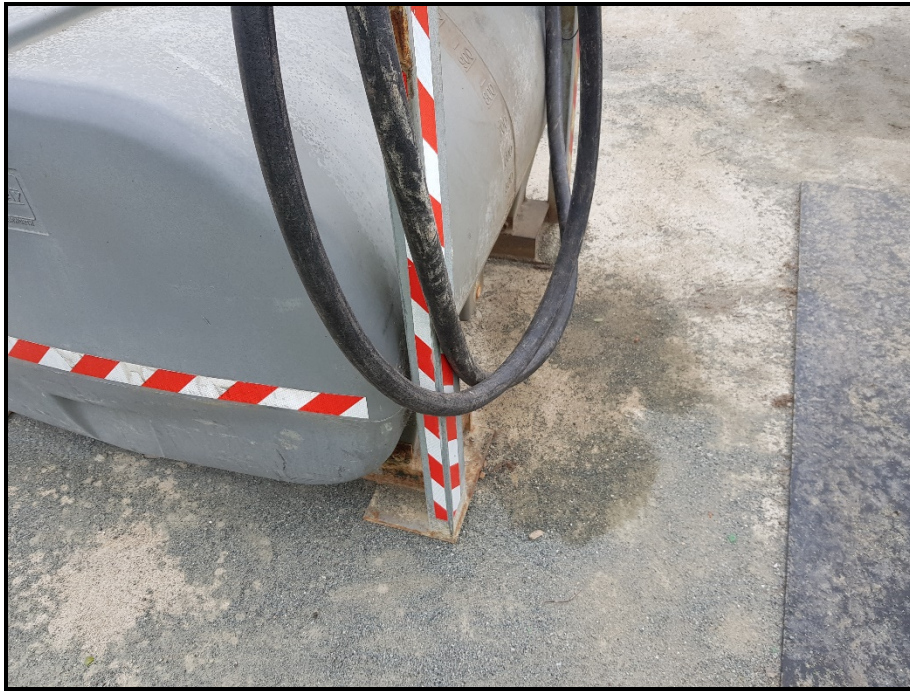
Photo 27: Unbundled, portable, grey Diesel tank (~1,000 L), reportedly empty with evidence of a minor spill from filling hose. 24/03/22
