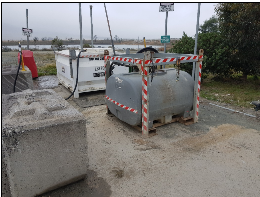
Photo 26: Self-bunded white Diesel tank (2,500 L) and unbunded, portable, grey Diesel tank (~1,000 L), reportedly empty. 24/03/22
