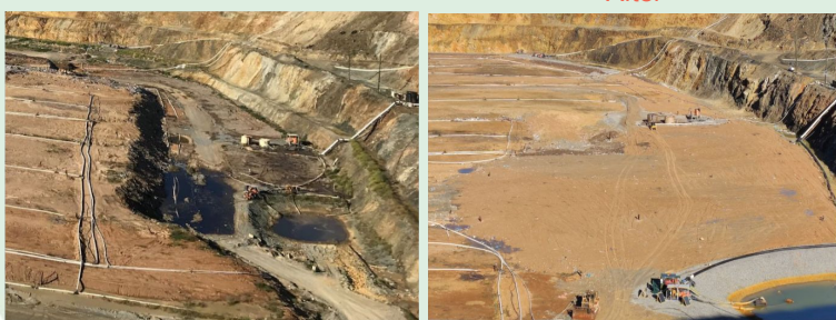
Before Western utility area After
