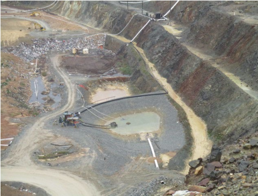
Figure B4. Photograph of the leachate treatment dam above the void.
