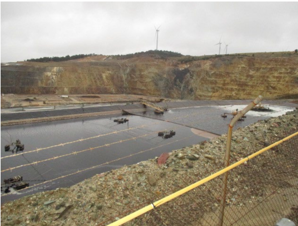
Figure B4. Photograph of the leachate treatment dam above the void.
