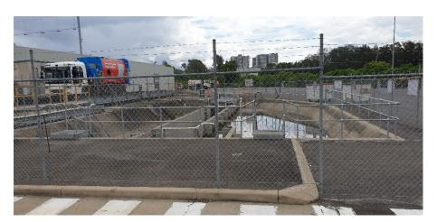
Plate 3: First flush stormwater system
