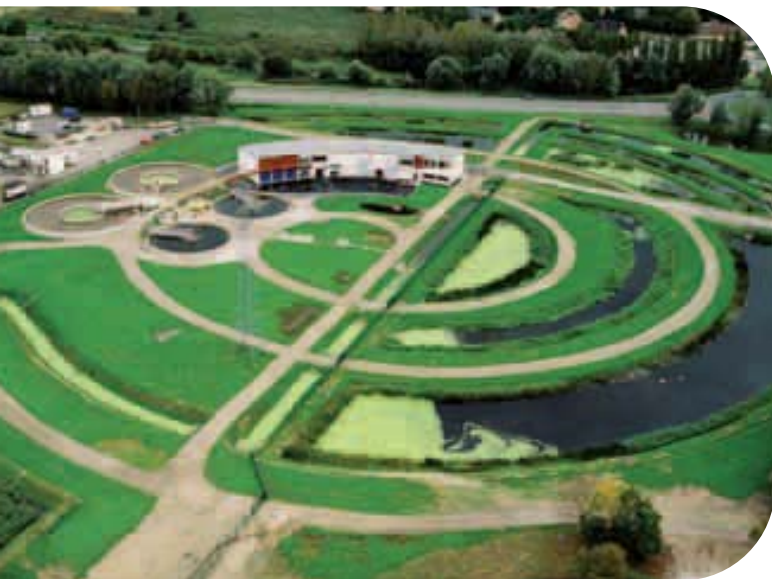
Aerial view of a Filtration Garden
