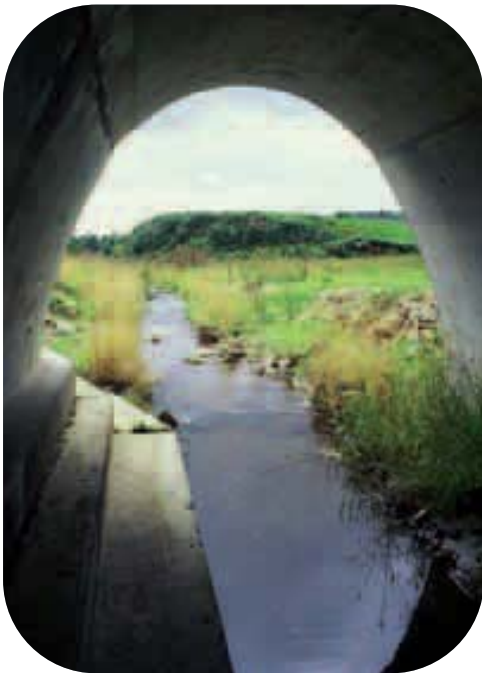
Artificial waterway for otters on motorway A89
