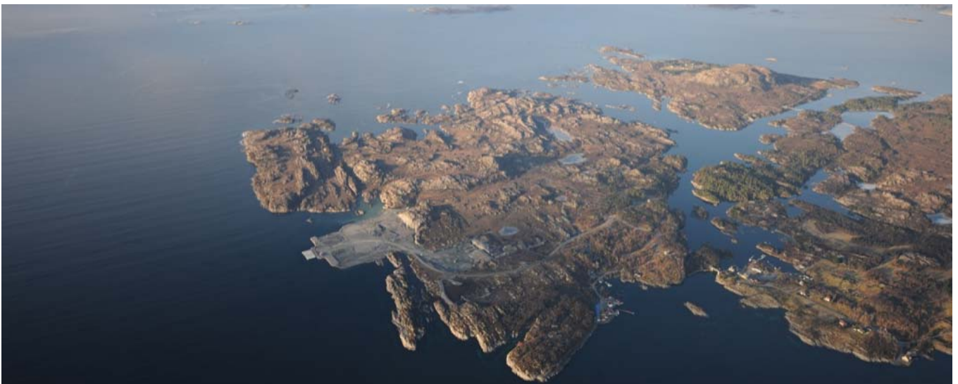
Veolia's decommissioning site in Lutelandet - Norway
