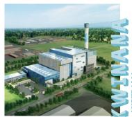
Australia's first waste-to-energy facility, the new Kwinana plant near Perth, will produce 40 MW of green energy – the equivalent of the consumption of 50,000 homes. This environmentally friendly solution will provide the city with a local, economical and secure source of energy. By 2021, the plant will process 400,000 metric tons of waste per year.
