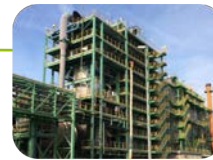
Rotating kiln incinerator
