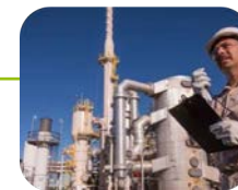
Sulfuric acid regeneration
