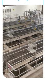
LEAPfas™ granular activated carbon and ion exchange lead-lag vessels
